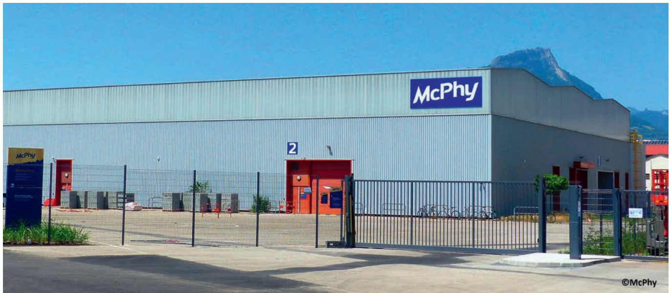
New McPhy site in Grenoble, bringing together Station activities and some head office functions.
