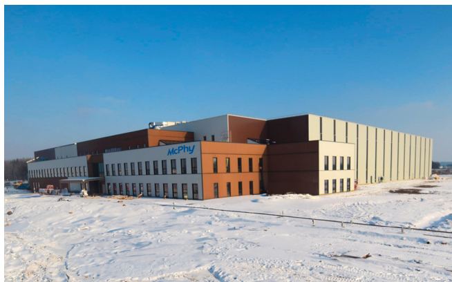
Site McPhy de Belfort (France)
